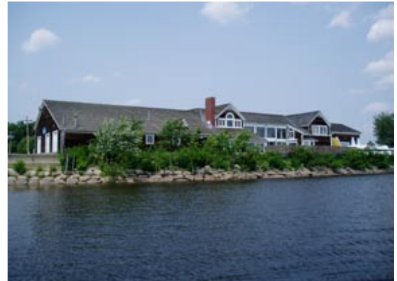
“The Boat House” at Regatta Field is a recreational amenity that is in need of major repair and preservation.
